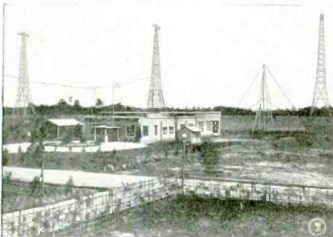
Fig. 3, above—Here we have an interesting view of the building housing the Receivers and auxiliary equipment for the short-wave phone service to America and located at Komuro, Japan. The antenna arrangement is supported by the masts shown, which are somewhat lower than those used for supporting the transmitting aerials. Fig. 4, to the right, shows Japanese engineer tuning one of the 20 kw. short-wave phone transmitters at Nazaki.
